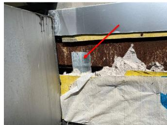
**IMAGE 1.15: METAL STRAPS USED TO ANCHOR SHEATHING**
