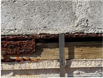
IMAGE 1.5: CORRODED STEEL
