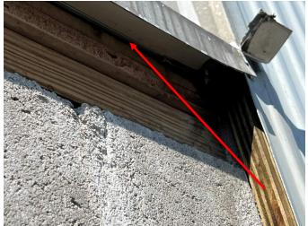
**IMAGE 1.4: MISSING WINDOW SEALANT**
