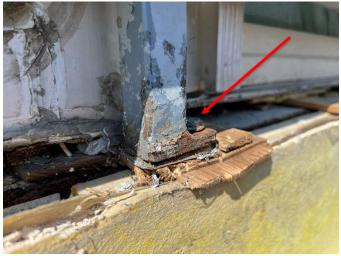
**IMAGE 1.12: RAILINGS ANCHORED TO SHEATHING**
