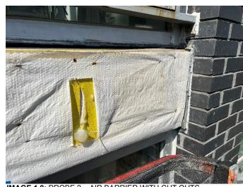
IMAGE 1.8: PROBE 2 – AIR BARRIER WITH CUT OUTS
