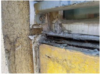
IMAGE 1.11: PROBE 2 - MISSING WINDOW SEALANT
