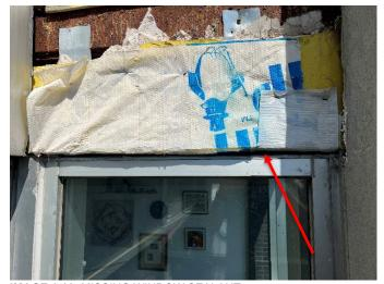
**IMAGE 1.16: MISSING WINDOW SEALANT**
